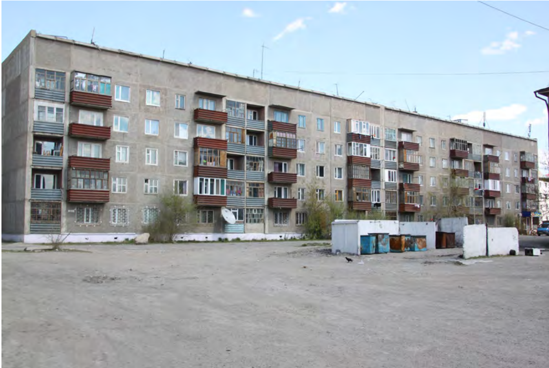
Figure 3: Apartment blocks . Photo credit: Author.
